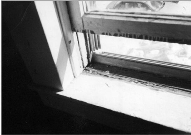
**A window well with deteriorating lead paint — a common site for lead poisoning.**
